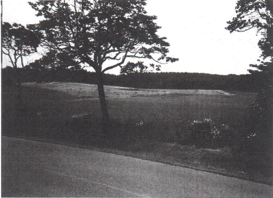
From Hammertown Lake Road looking west at excavated site (1997)
